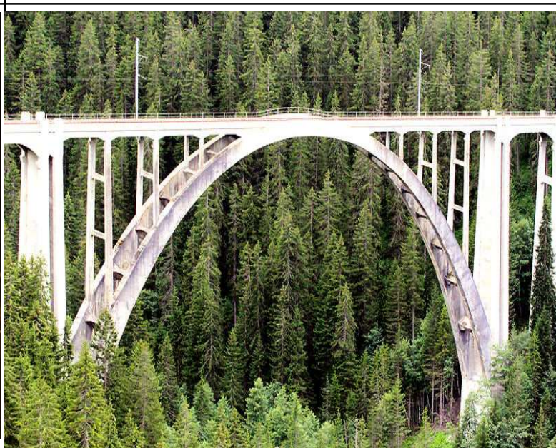
Langwies viaduct on the RhB Arosa line, Switzerland
